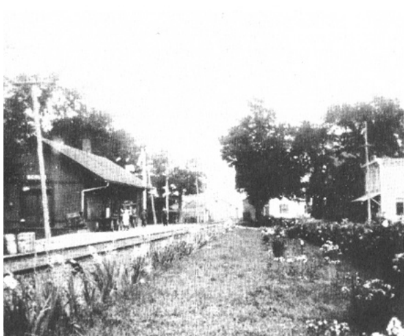
The track side of the Berlin Station shows us the loading platform with milk cans and passengers awaiting the next train. With Arthur Cowee's interest in gladiolus and hydrangeas, we assume that he was responsible for beautifying the station yard. The building on the right was Porter Lamphier's Store.
