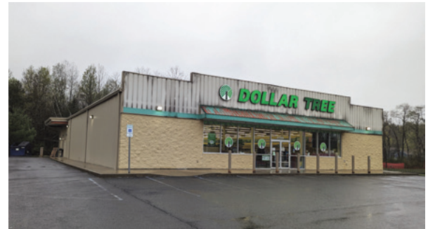
The former Dollar Tree on State Route 22 in Hoosick Falls, which the county is seeking approval to purchase in order to convert it into a Senior Center, DMV satellite office, and mental health counseling services center. Photo courtesy of Rensselaer County.
