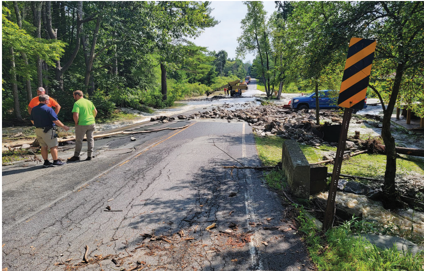
The aftermath of a flood caused by a dam break in the area of Garfield Rd on the morning of July 24th. Photo courtesy of the Stephentown Volunteer Fire Dept.
