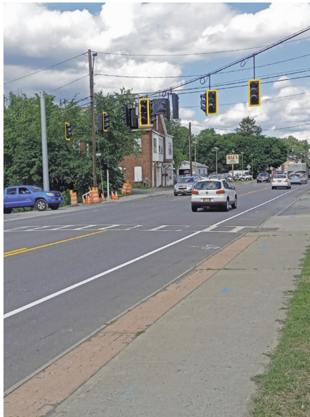
The traffic signal installed by the NYS Department of Transportation on Hoosick Road at the intersection with Lord Avenue hangs above the roadway, just waiting to be energized. Photo by Doug La Rocque.
